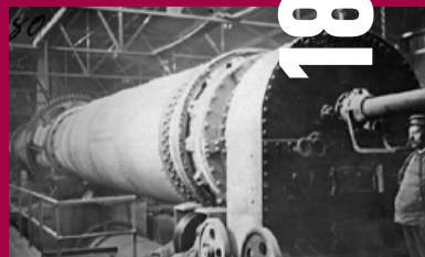
The American rotary kiln, invented by Aalborg Portland's Poul Larsen, built for the first time in Europe, as two new rotary kilns are installed at the Rørdal factory. The production capacity is significantly upgraded.
